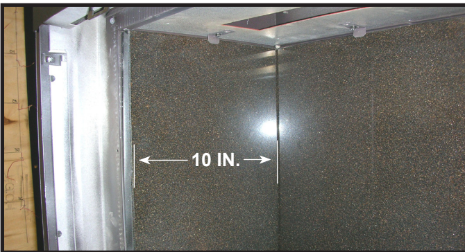
Figure 8. View of Back and Side Piece Installed.
